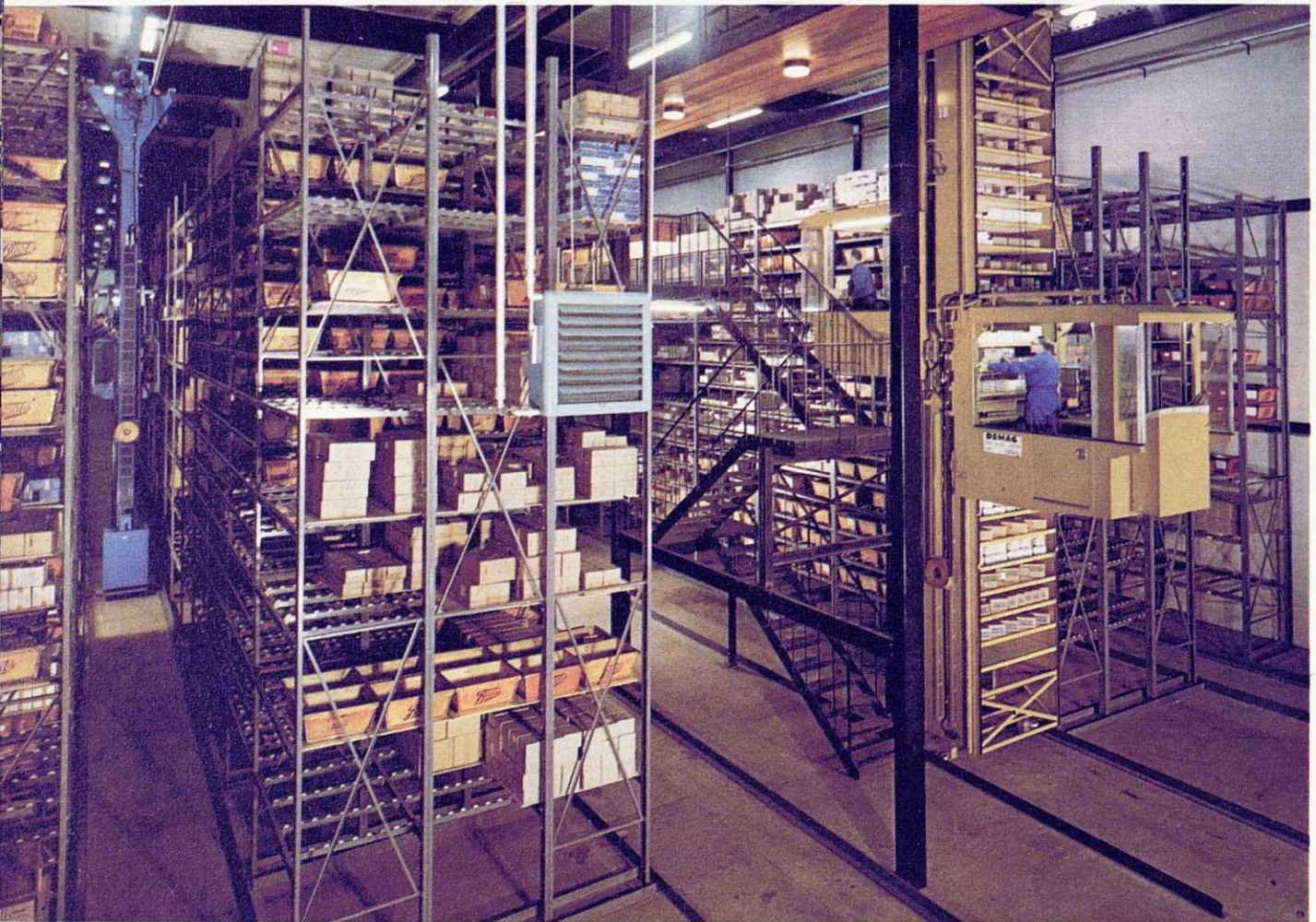
Top Left: Part of the new Insulin manufacturing plant. Top Right: A new soap drying plant. Below: The new automated warehouse for toilet merchandise. On the right of the picture two operators in moving cabs can be seen picking the merchandise.
